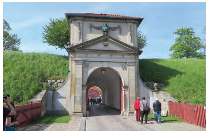
The impressive Kings Gate – the main southern entrance to Copenhagen castle (Kastellet), dated 1663. The bust is of Frederik III
